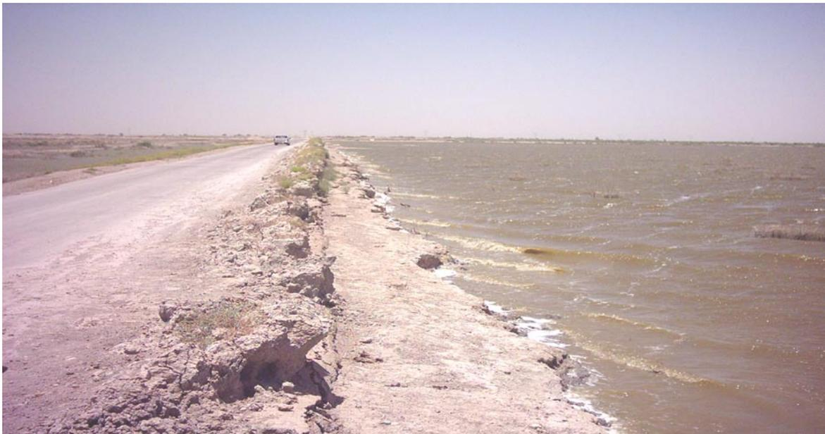
Figure 30: Dyke with roadway separating reflooded and unflooded zones.
